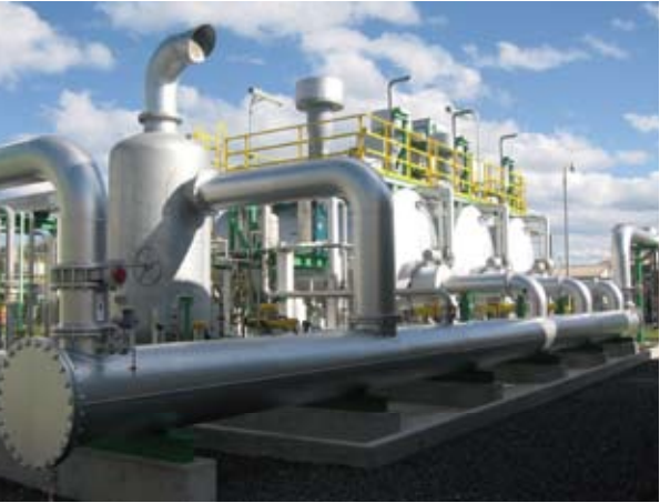
Equipment for recovery of solvents from discharged gas
